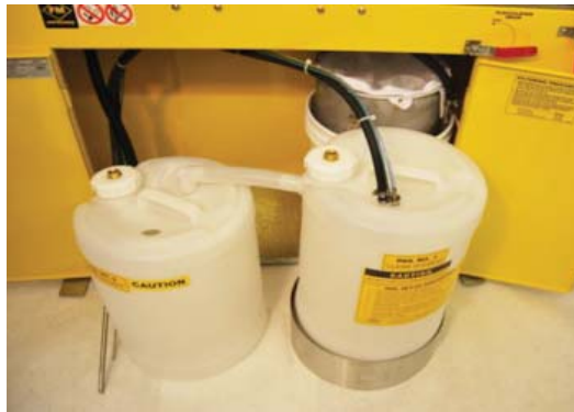
Left and center pails can be connected to a Uni-ram recycler (UG5000EW only)
